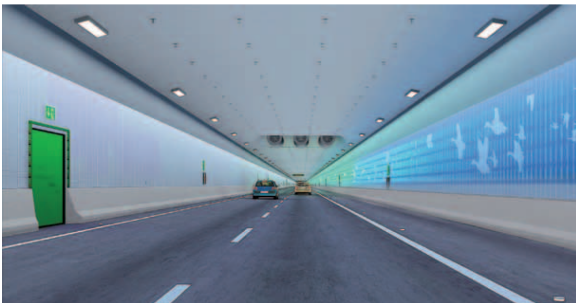
Figure 7. Three colored zones and illustrations on the walls of the road tunnel will help to give motorists a varied journey during their 10 minute drive through the Fehmarnbelt tunnel.
